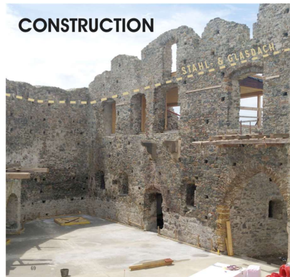
Figure 4a, Unrestored Taggenbrunn castle courtyard, yellow line indicates the future position of the transparent glass coverage
