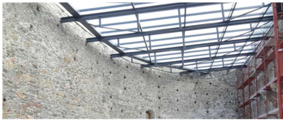
Figure 4b, Taggenbrunn castle courtyard transparent glass coverage
